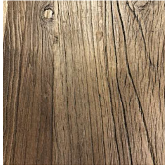
Small cracks along grain lines
